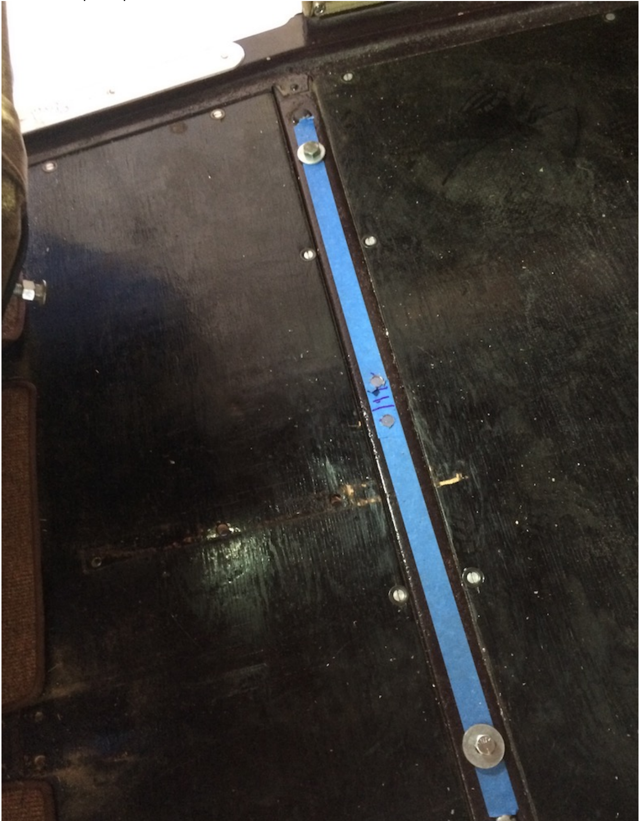
Closeup of tape on floor where bolts will be drilled
